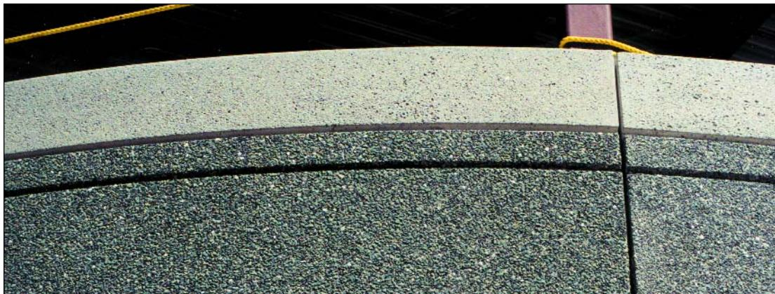
show any obvious imperfections other than minimal colour and texture variations, nor should it provide evidence of repairs when viewed in typical lighting with the unaided naked eye at a 6 meter viewing distance. Appearance of the surface should not be evaluated when sunlight is illuminating the surface from an extreme angle, as this tends to accentuate minor surface irregularities.
