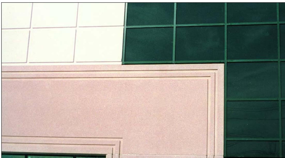
be controlled within the limits of strength and absorption requirements and not exceed 6% by weight of cement. Different shades of colour can be obtained by varying the amount of pigment or by combining two or more pigments. White Portland cement will produce cleaner, brighter colours and should be used in preference to grey cement, especially for the light pastels such as the buffs, creams, and ivories, as well as the bright pale pink and rose tones.
