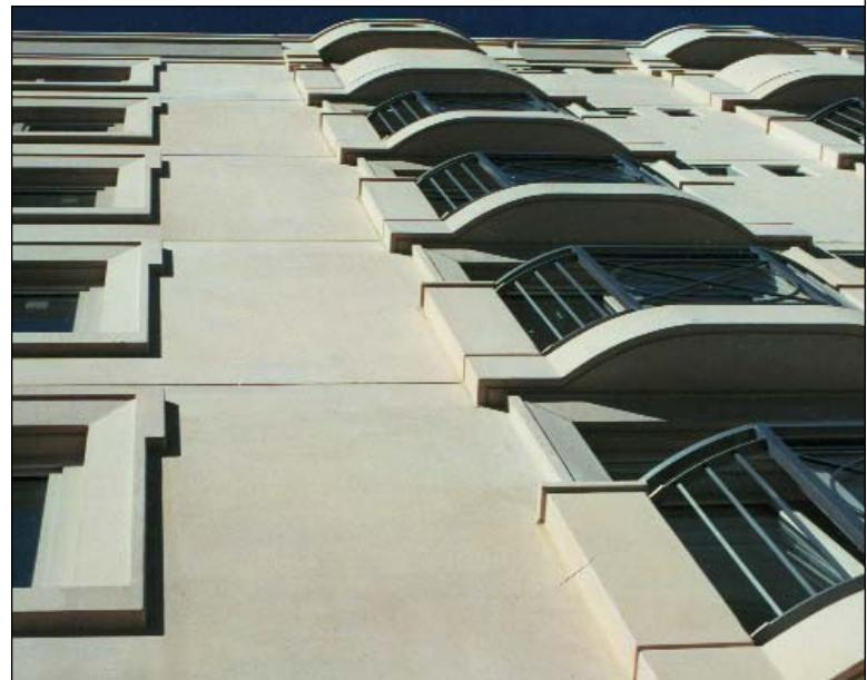
It is important to select appropriate aggregates for this type of finish, aggregates which are acid resistant (siliceous type aggregates) whereas softer aggregates such as limestone and marble will be adversely affected by exposure to acid.
